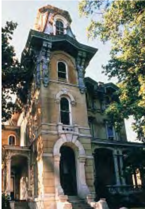
The Fontaine House, built 1870 in the French Victorian style.
